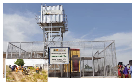
Completed 5000 gallons Solar Hybrid System Powered Water, Sanitation and Hygiene facility provided by NNPC/SNEPCo as part of its humanitarian intervention in Kwaya Local Government Area of Borno State. Project was completed in 2020 serves over 11,450 people resident in Kwayakuser community.
